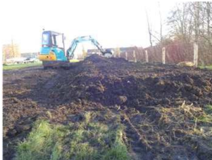
Above: Final round of mixing, leveling and mound making
