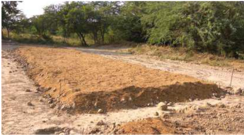
Biomass Spreaded On Top Layer
